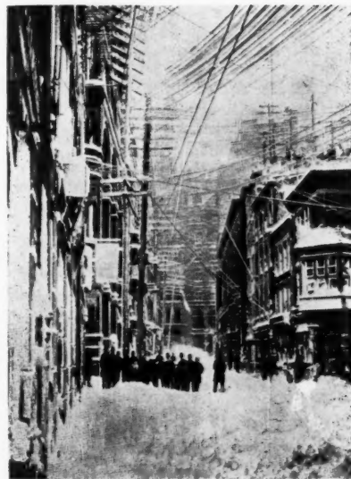
New Street, N. Y., after the storm. Every one of New York's 6,000 telephones went dead; telegraph communication to Boston and Washington was by way of cable to London.
